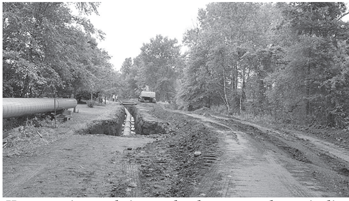
Heavy equipment being used to bury natural gas pipeline.
