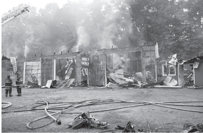
Fire leveled the Herrick Township Municipal Building on Tuesday.
