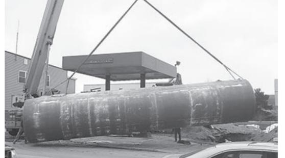
A large crane and excavating equipment were used to remove the gasoline tanks from Hornbeck Chevrolet on Main Street in Forest City last week. It took a few days to complete the project.
